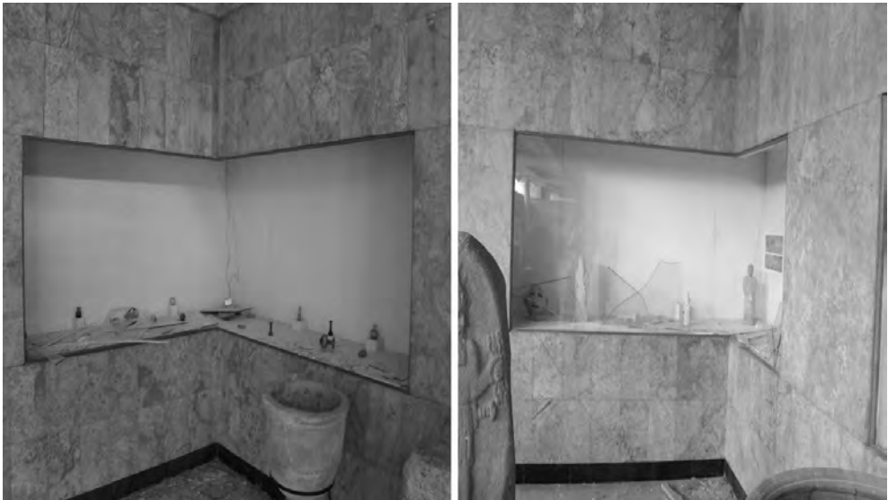
Fig. 2. The damage inside the Classical section of Aleppo Museum (the objects on display are copies).
