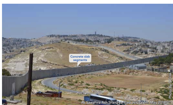
(a) Concrete barrier
