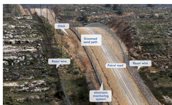
(b) Chain-link barrier
